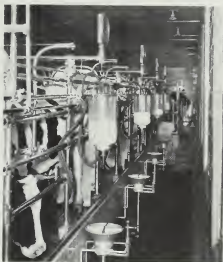
The new cow barn with places for 100 animals; on the left is the milking house; center foreground, pens and stalls for the two bulls; below, the milking stalls and electric milkers
